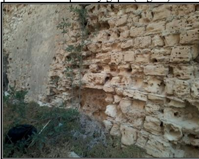
Figure 22: A model of the gaps of dissolution in the western façade of the southern tower of Kousa Pasha Fort
