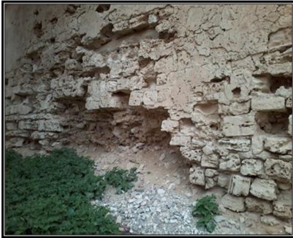
Figure 24: A model for Granular disintegration in the eastern facade of the northern tower, Kousa Pasha Fort.
