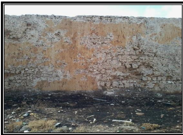
Figure17: A model of mortar fall of Kousa Pasha Fort.
