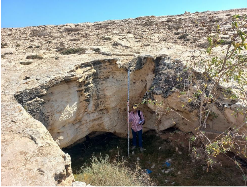
Fig. 10: A collapsed sink hole near the lighthouse, with the edges trimmed for housing or grain preservation.
