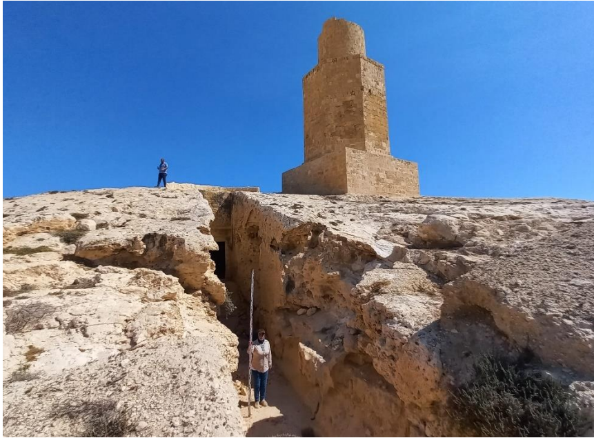
Fig. 15: Entrance to the tunnel dug below the limestone ridge; it starts from the southern slopes overlooking Lake Mariout to the shore of the Mediterranean Sea, with a length of about 1.3 km.
